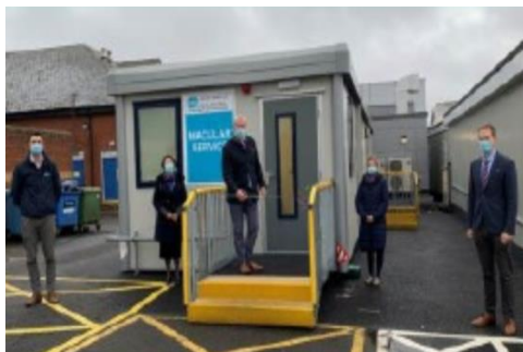
December 2020: The opening of the new Modular Building for the Macular Service at Musgrave Park Hospital
